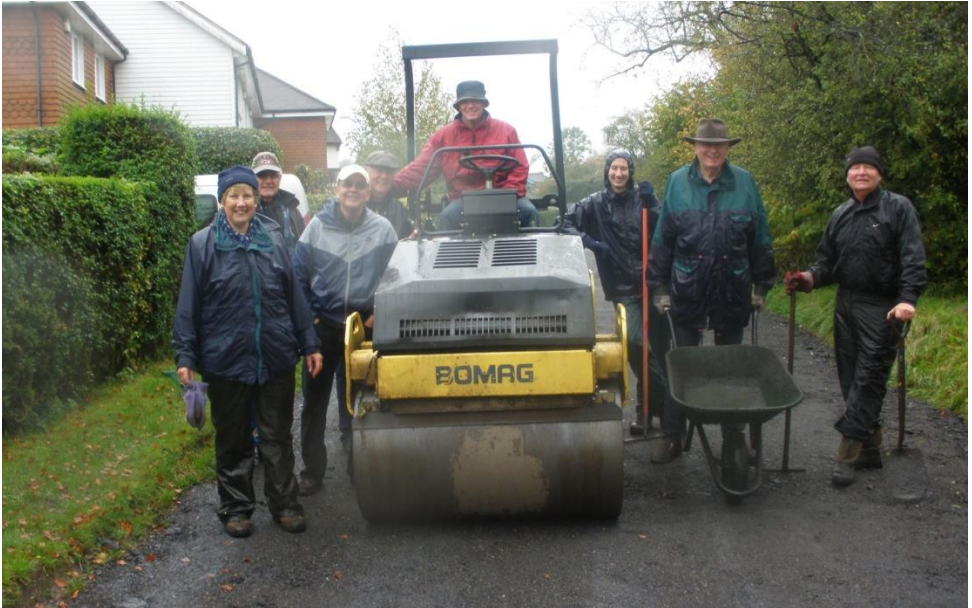
A little rain does not deter the residents of Johns Road from making life run more smoothly – see page 23
